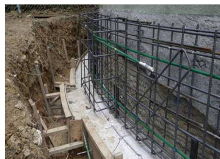
補強後：周壁を増厚補強
